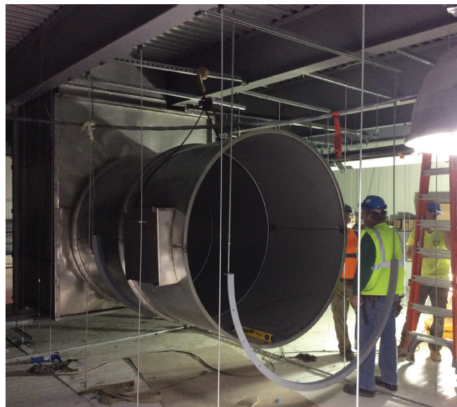
Sheet metal workers installing some 76" stainless steel supply duct, at the Kraft-Heinz Plant Expansion in Lowville, NY, one of Hyde-Stone's currently ongoing projects. Photo by Chris Stone.
