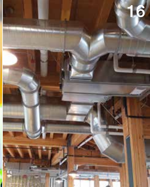
Photo courtesy of Auburn Mechanical
