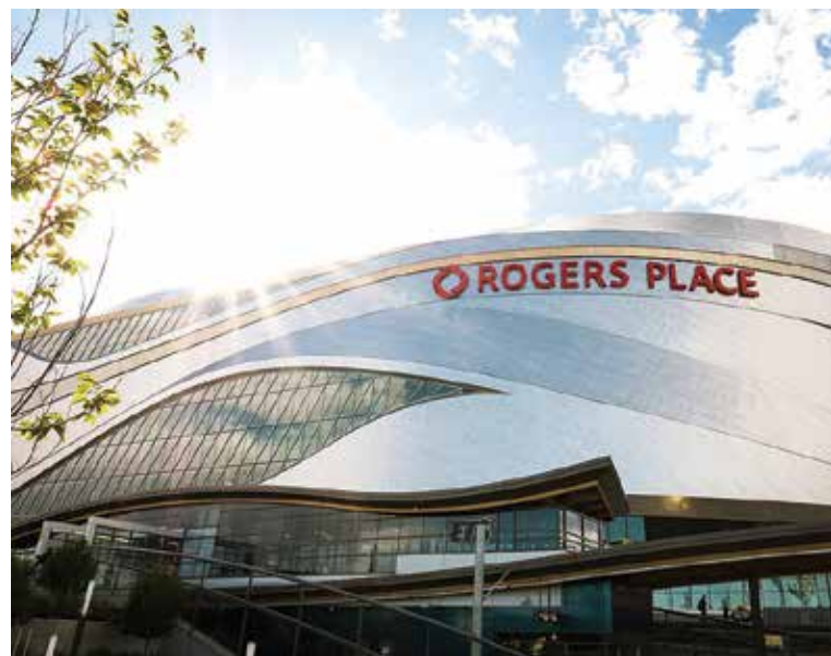
Rogers Place in Edmonton | Photo: Western Mechanical Services
