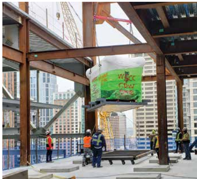
Prefabricated condenser water pump skids hoisted into position on level 12.
