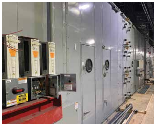
Installation in-progress of 1 of 35 air handing units. • Photo by Gus Simonds
